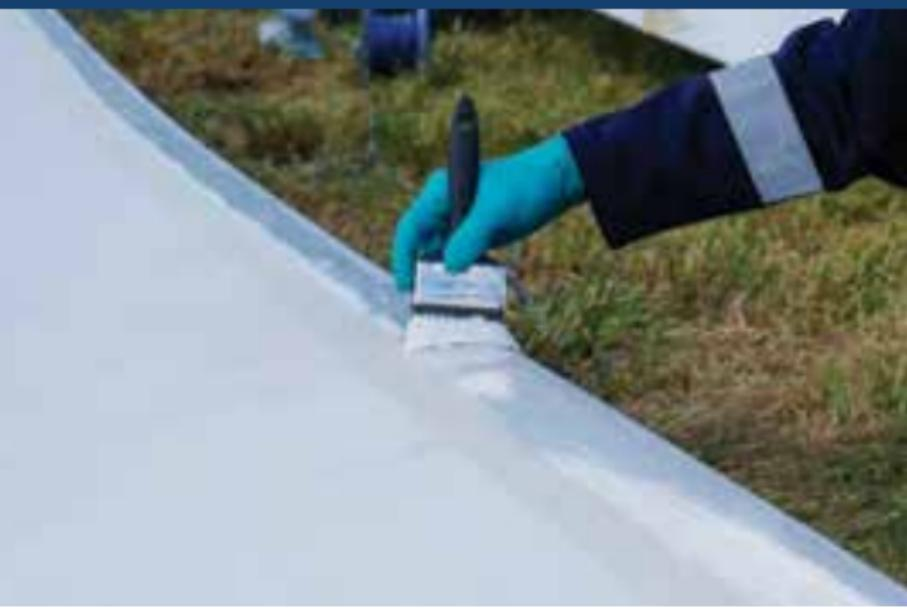
Materials for rebuilding and protecting the leading edge of wind turbine blades from erosion.
