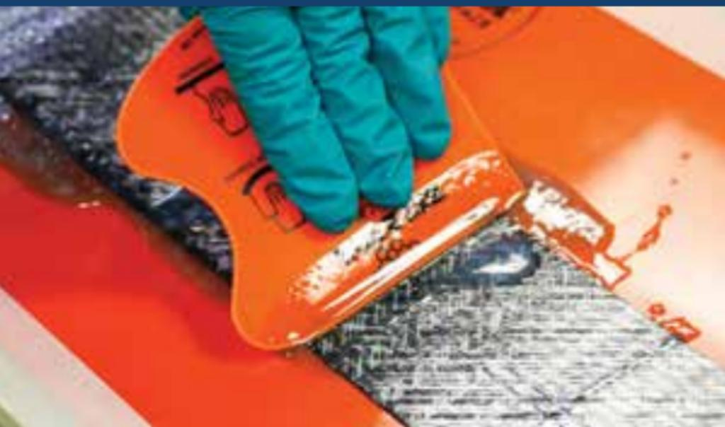
Thermoset resins reinforced with fibers and tested as a repair system to the requirements of internationally recognized standards.
