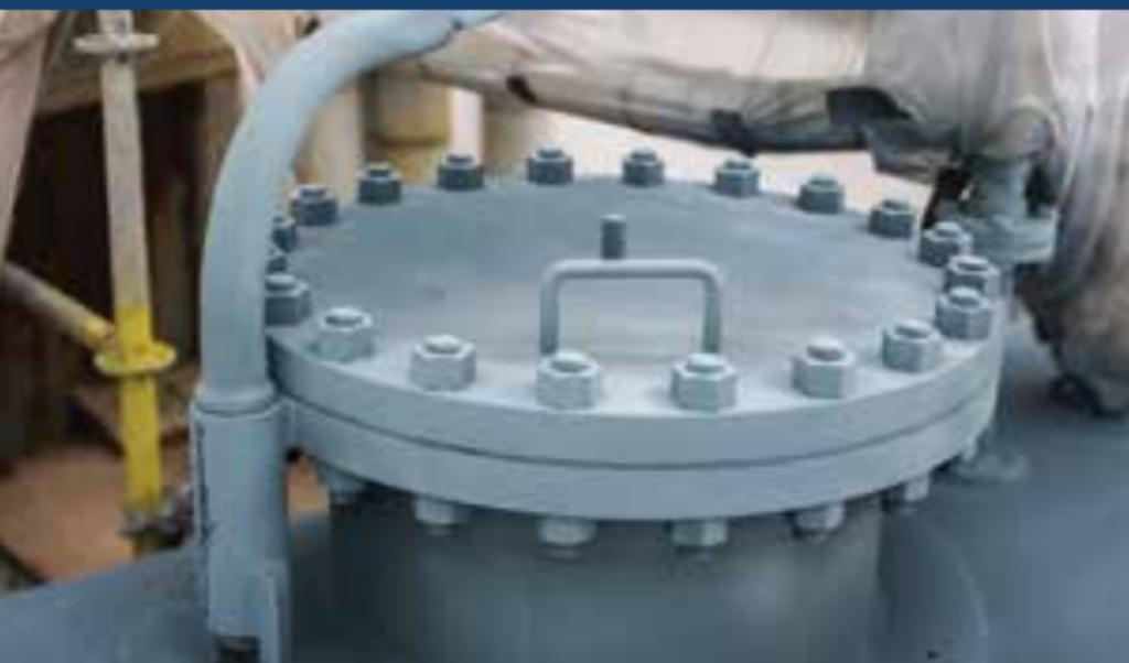
Zinc-rich epoxy materials for corrosion protection to steelwork.
