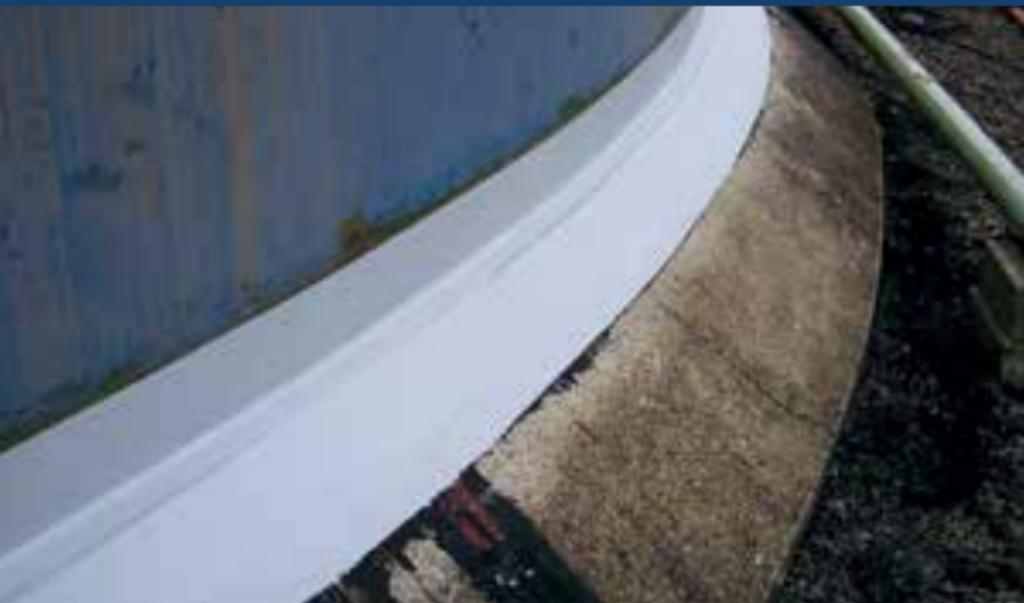
Waterproofing and fire-resistant membrane for the protection of insulation and cladding materials.
