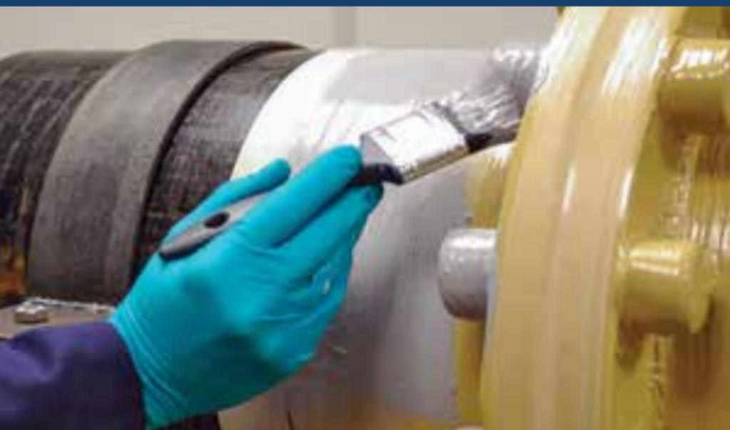
Peelable encapsulating system for protecting pipework and other structures from external corrosion.
