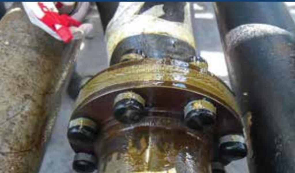
Corrosion inhibiting material with releasing properties.
